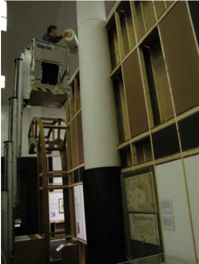
Above: Head of Exhibitions, Alan Sterenberg, installing a roll of fire-retardant fabric above a 16th century Belgian tapestry
